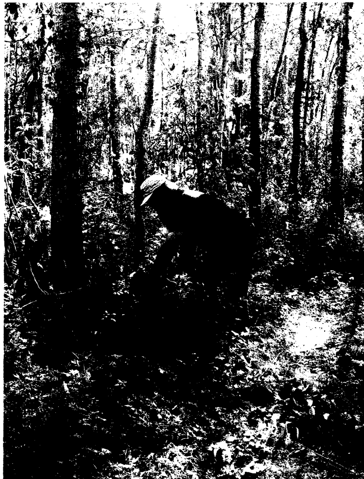
Removing stumps and roots before installing road cloth
