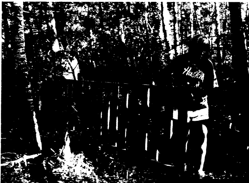
The major components were prebuilt
